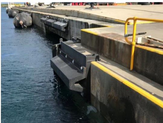
Installed fenders on the southern side of the wharf.
