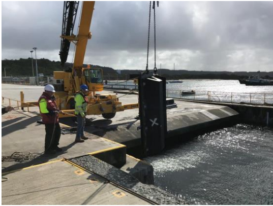
Installing the new fenders
