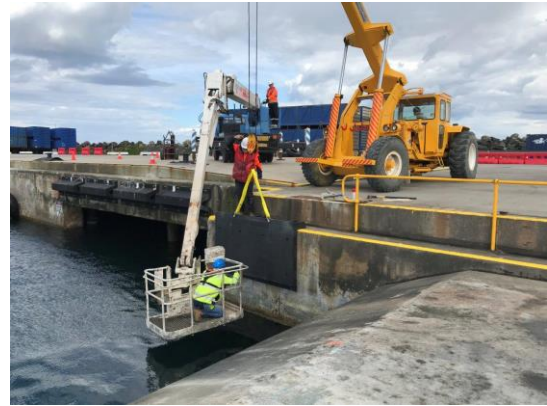
Installation of new fender brackets
